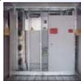
2 Supply air mixes with return air.
